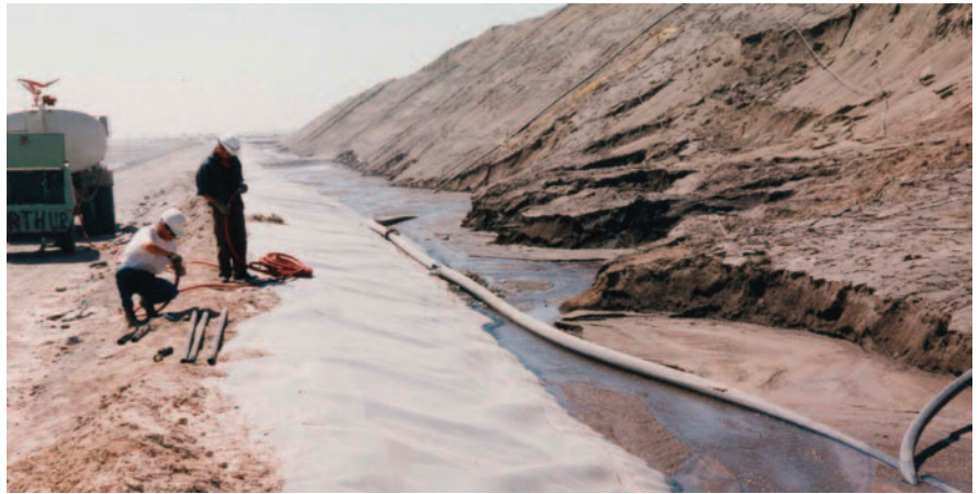
Example of a poorly performing heap leach facility. Photo shows sloughing of heaped materials due to elevated fluid levels within the heap.
