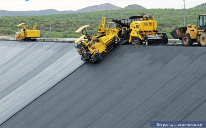
he Sartorius Von Bach Dam (Von Bach Dam), situated east of Okahandja in Otjozondjupa Region, has recently received a new bituminous seal layer after approximately 50 years of service. The previous asphalt seal had become brittle, due to loss of volatiles from the bitumen, which typically leads to cracking on the surface of the asphalt.
