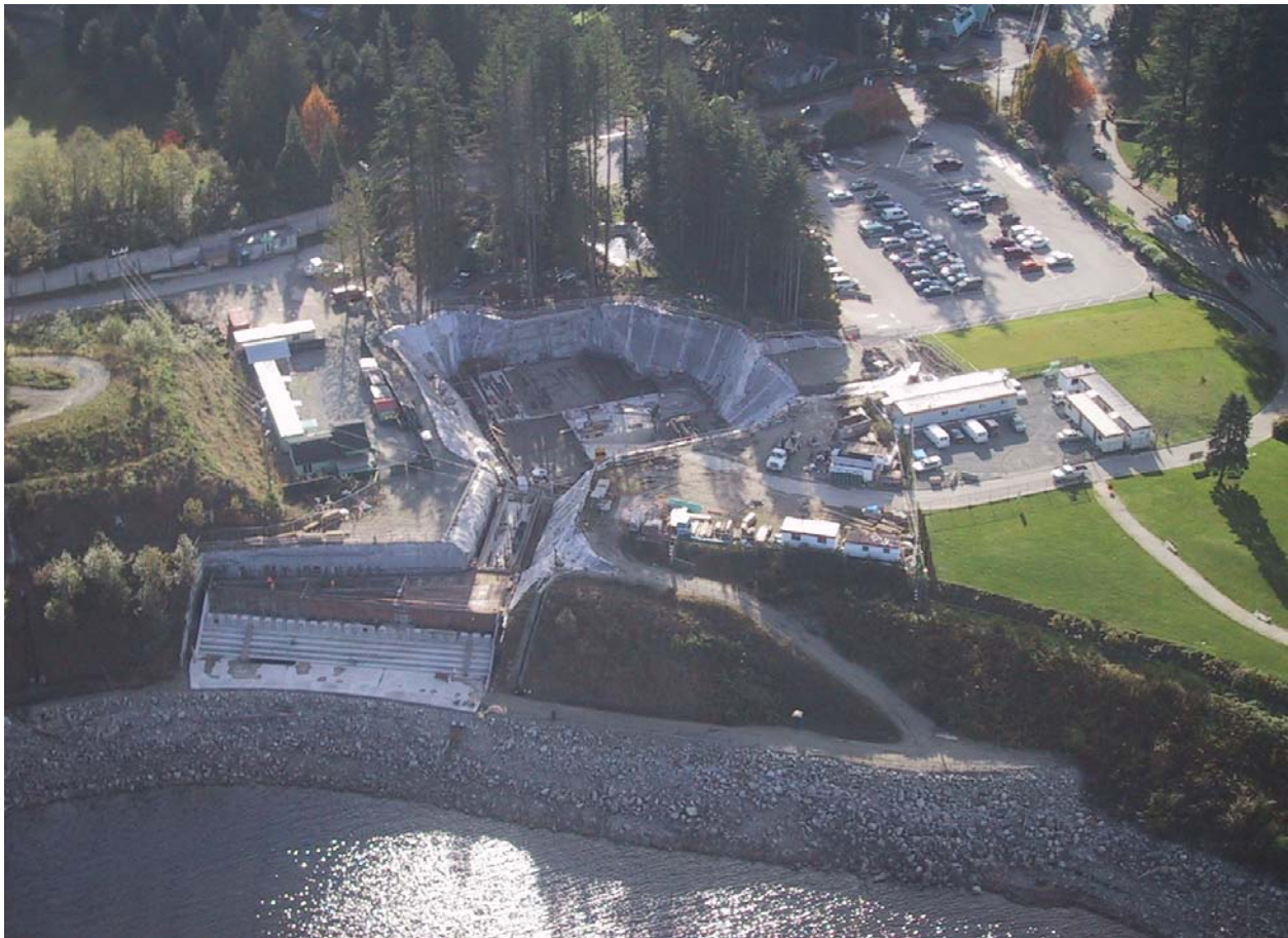
Figure 6: Excavation during construction. Note overflow channel and spillway
