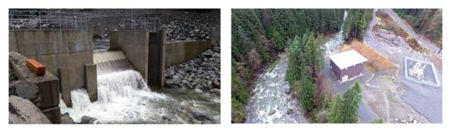
Figure 1: Marty Creek intake (left) showing the Coanda screen intake and side-spill weirs. Powerhouse and substation (right) adjacent to McNab Creek.
