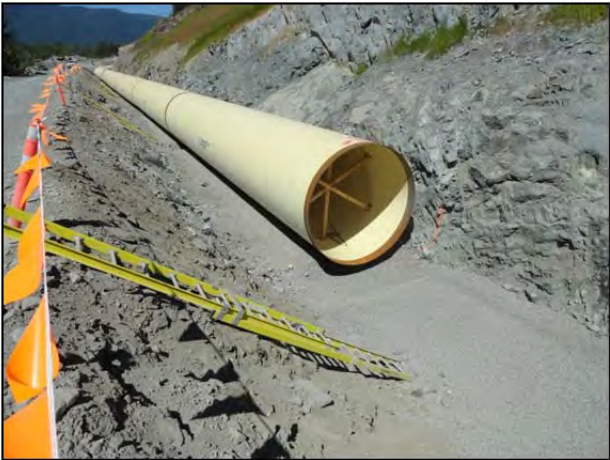
Photo 10 – Penstock Pipe Placement
