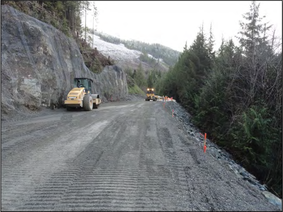
Photo 12 – Penstock in Road Section Construction
