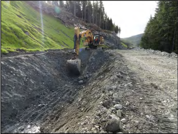
Photo 9 – Penstock Trench Excavation
