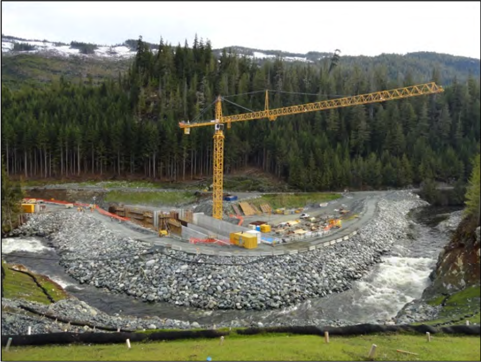
Photo 4 – Temporary Diversion Channel During Construction of Intake
