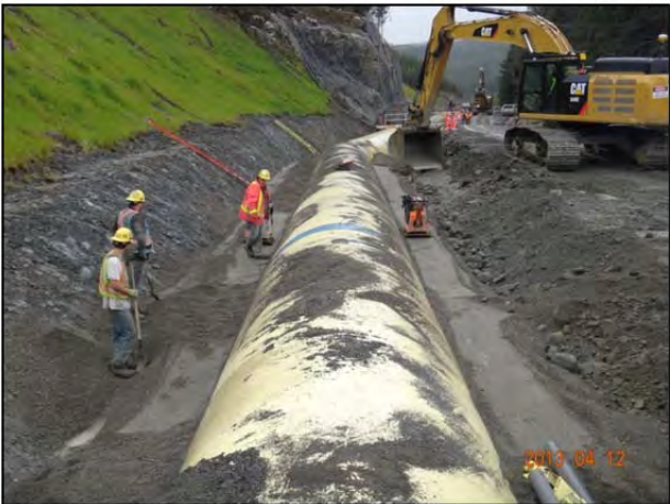
Photo 11 – Penstock Pipe Placement
