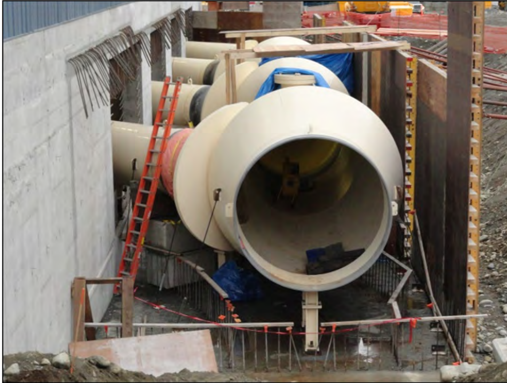
Photo 8 – Penstock Quadfurcation Manifold (under construction)
