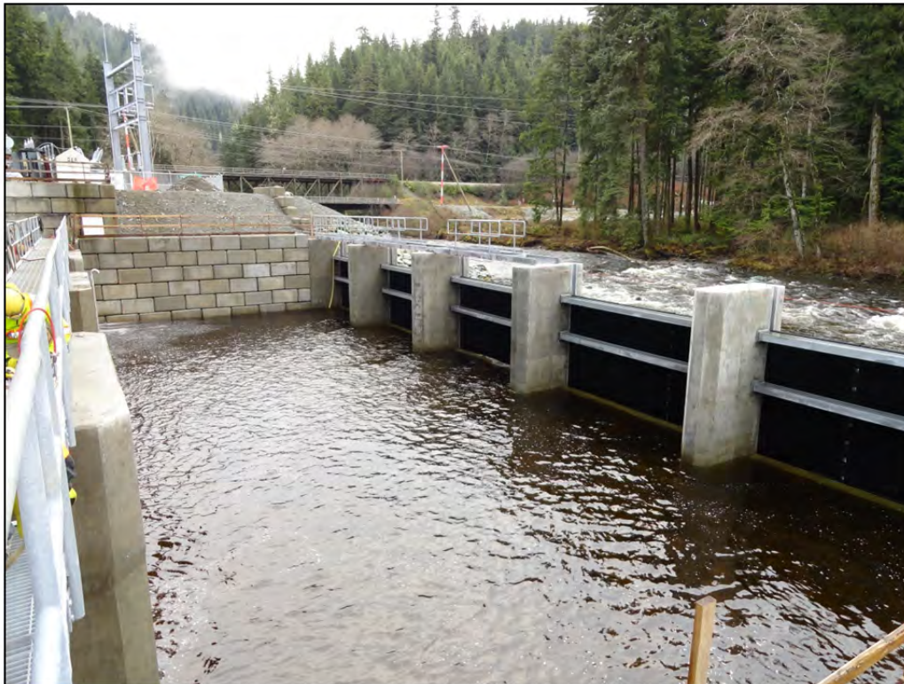
Photo 15 – Powerhouse Tailrace (back flooded)
