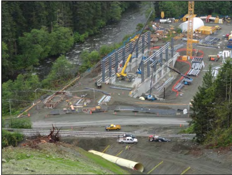
Photo 14 – Construction of Powerhouse, Switchyard and Penstock
