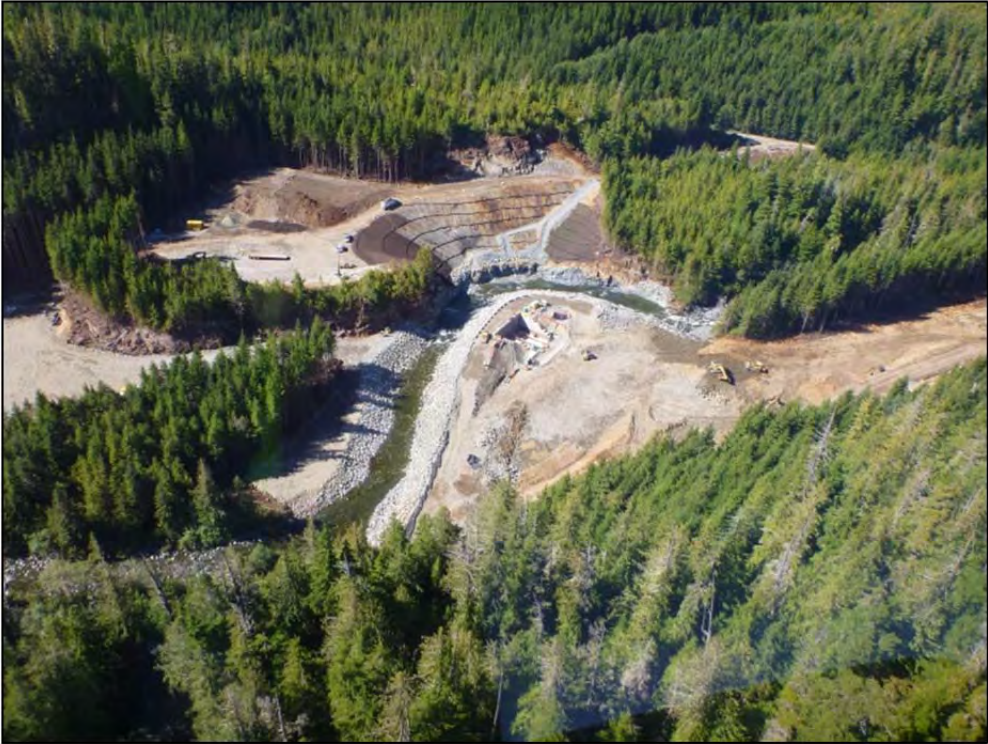
Photo 3 – Temporary Diversion Channel
