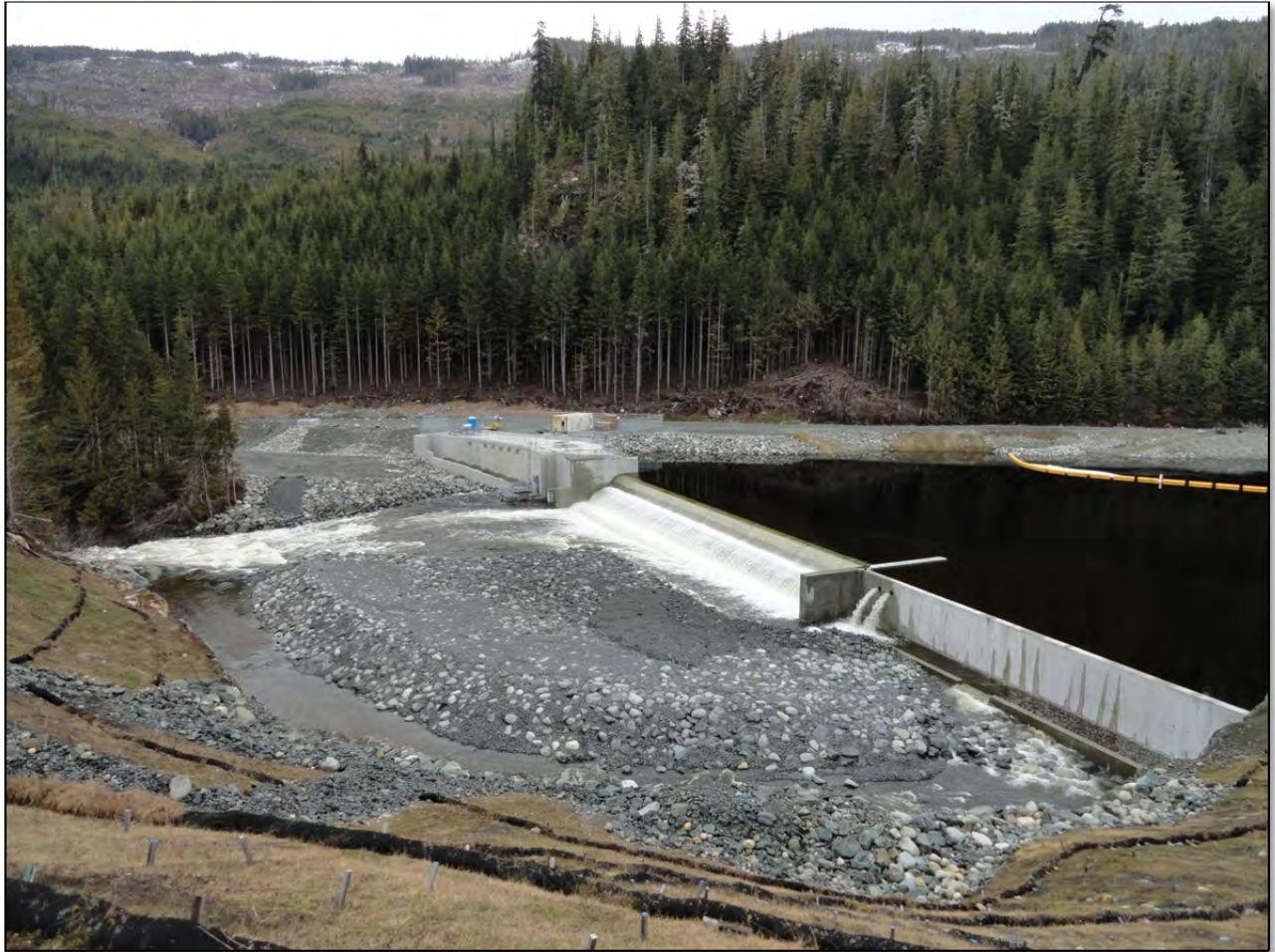
Photo 1: Kokish River HEP Headworks
