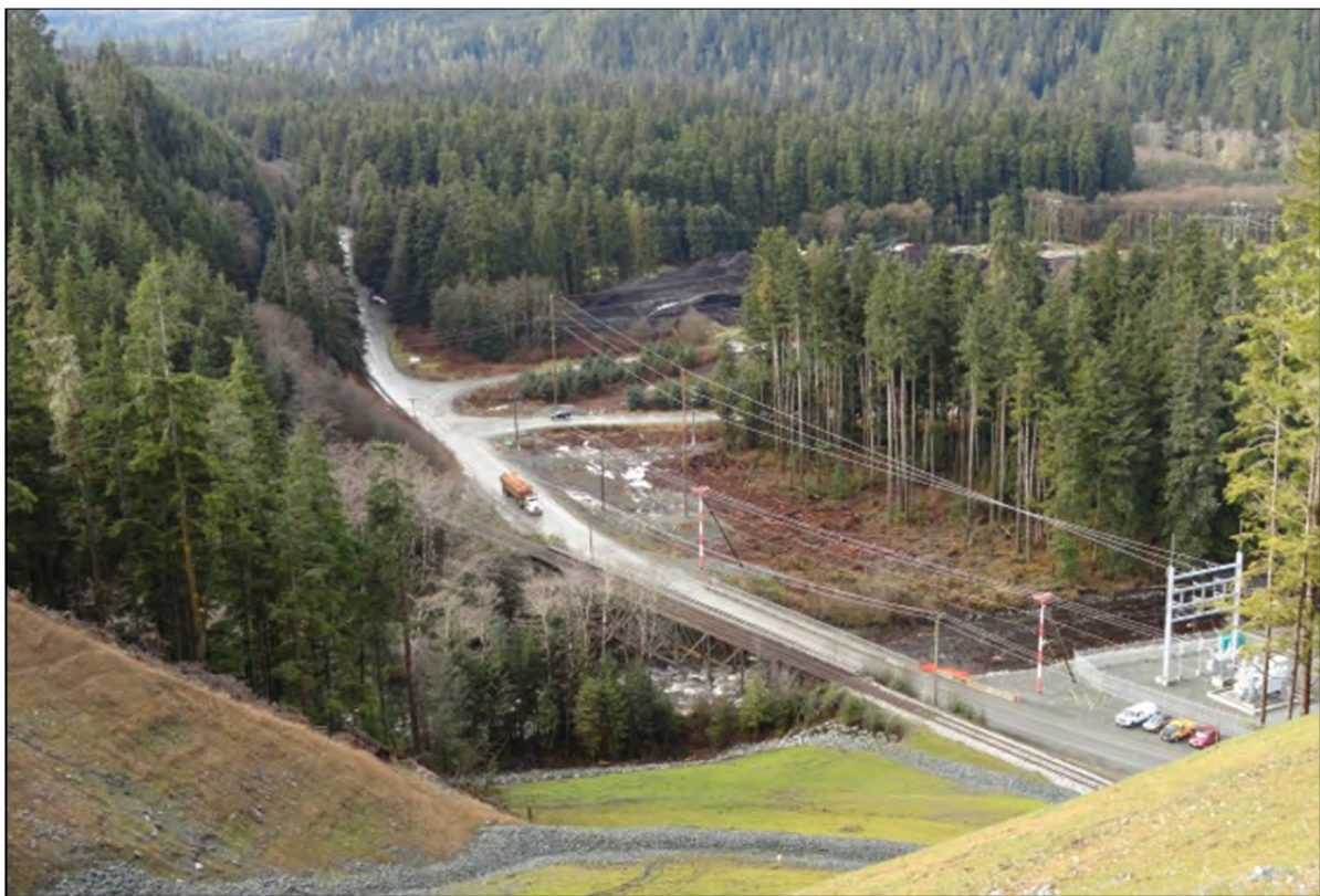
Photo 18 – 138 kV Transmission Line
