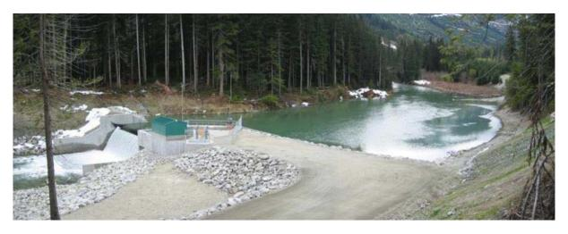
Figure 2. Rutherfod Creek 49 MW Hydro Project - Inflatable Rubber Dam
