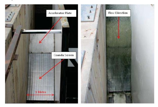
Figure 6. Full Scale Coanda Screen Model
