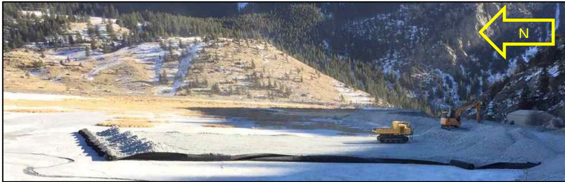
Figure 5 Closure Cap – Initial Construction Progress
