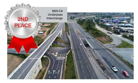
the C9 route to split away smoothly from the C3 route and loop back on itself, a viaduct for the continuing C3 route, realignment of an existing highway off-ramp and creation of a matching on-ramp, and, of course, the underpass itself, which connected the two highway ramps in a halfdiamond configuration.
