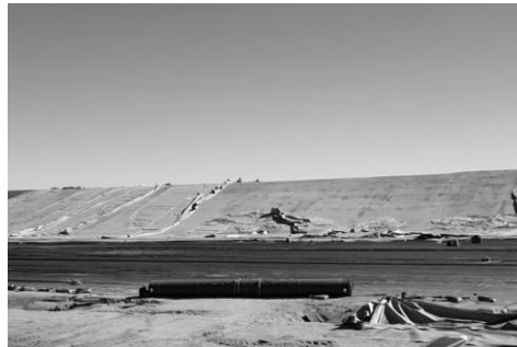
Figure 8. Newly opened (cut) starter wall
