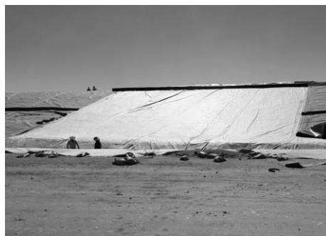
Figure 9. Re-placed geotextile with tacked edges
