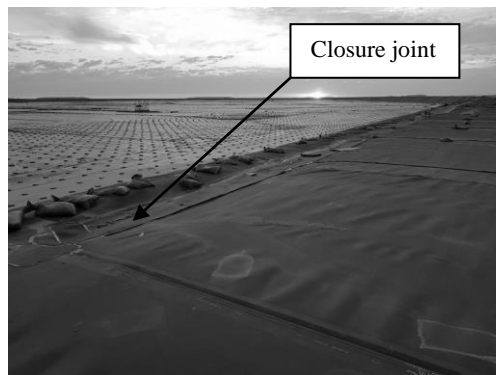
Figure 10. Crest on the starter wall being ballasted with sand bags
