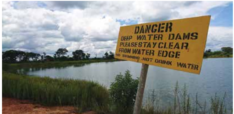
← Unlined pollution control dam at a copper mine
