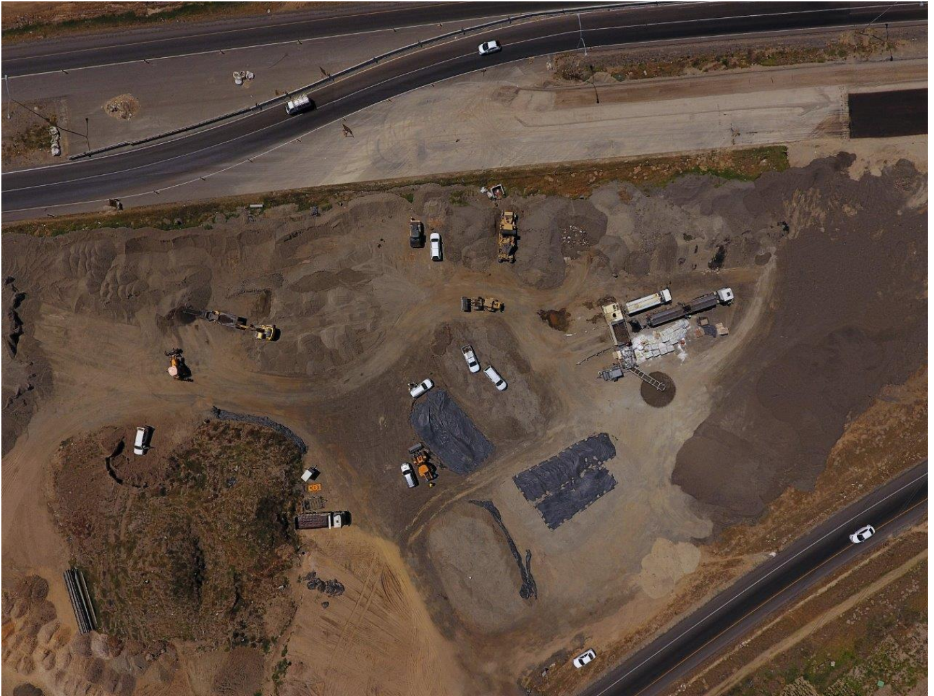
Fig. 6. Stockpile and BSM processing area at the Potsdam Interchange
