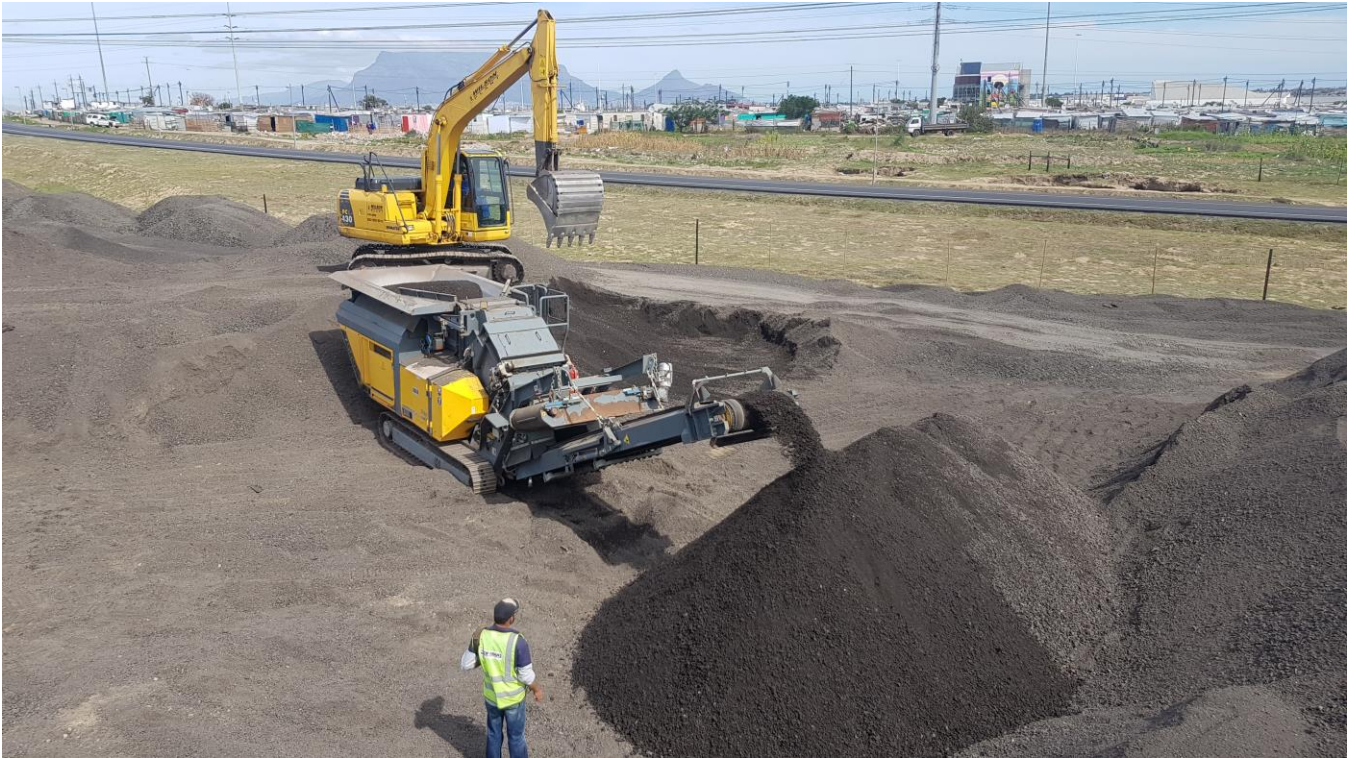
Fig. 5. Crushing the RA at the Potsdam Interchange
