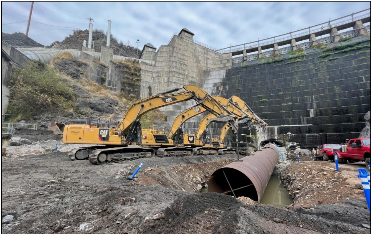
Figure 5: Copco No. 1 Dam with low-level outlet under construction, November 2023
