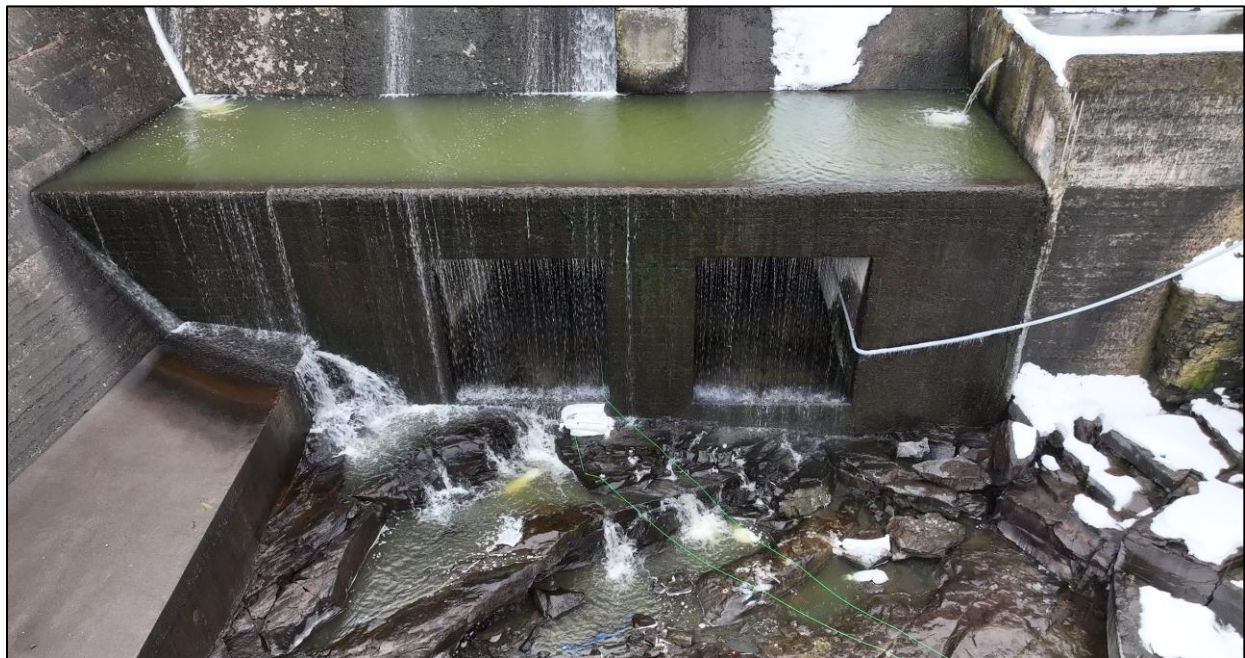
Figure 3: J.C. Boyle historic diversion culverts, prior to opening for drawdown initiation, January 2024
