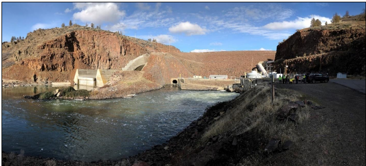
Figure 6: Iron Gate Dam, looking upstream
