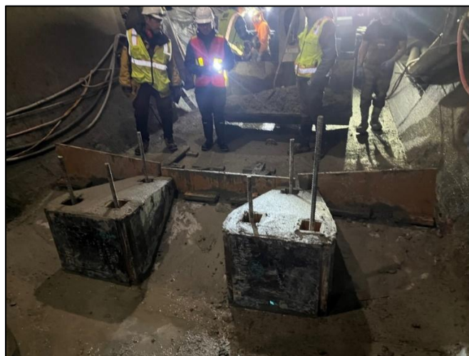
Figure 7: Iron Gate diversion tunnel – energy dissipation baffles under construction, December 2023
