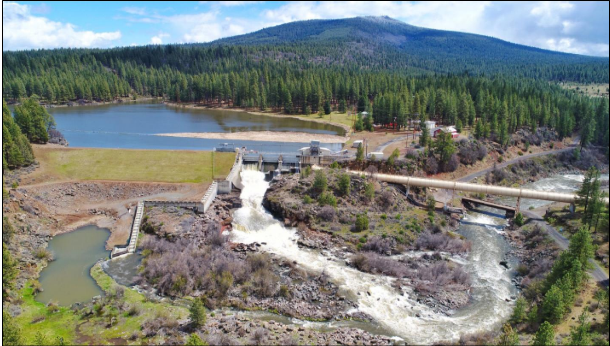
Figure 2: J.C. Boyle Dam, looking upstream (courtesy AECOM et al, 2018)
