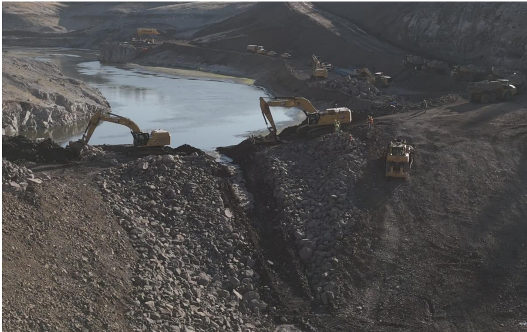
Figure 10: Final Breach of Iron Gate Cofferdam, August 28, 2024
