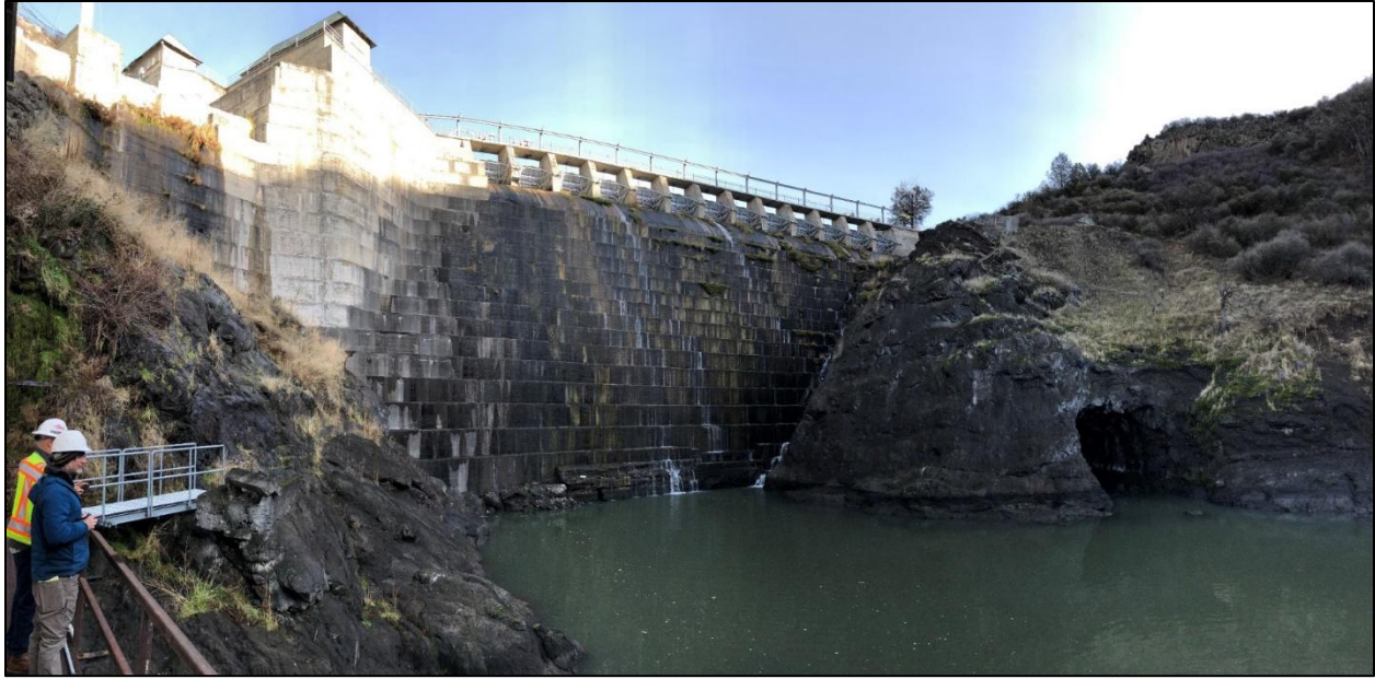
Figure 4: Copco No. 1 Dam and historic diversion tunnel, looking upstream
