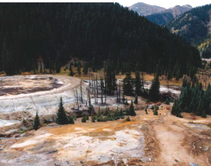
The Lead Carbonate Tailings Impoundment as it appeared before 1991 (left). The same area as it appeared in 1994 (right) after SGC relocated 27,000 yd 3 of tailings to Mayflower Impoundment No. 4, and regraded, neutralized and reseeded the area.
