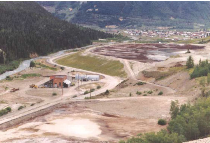
Before and After: Mayflower Impoundments Nos. 3 and 4 as seen in 1992 (left). SGC regraded the top of No. 3 (foreground), capped it with subsoil and reseeded it. SGC relocated 80,000 tons of waste to No. 4, regraded the area, and re-seeded it. This is how it appeared in 1995 (right).
