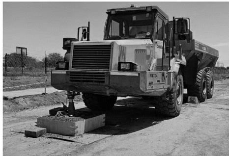
**Fig. 2.** Test pad under construction to monitor damage and strain in the Geomembrane.
