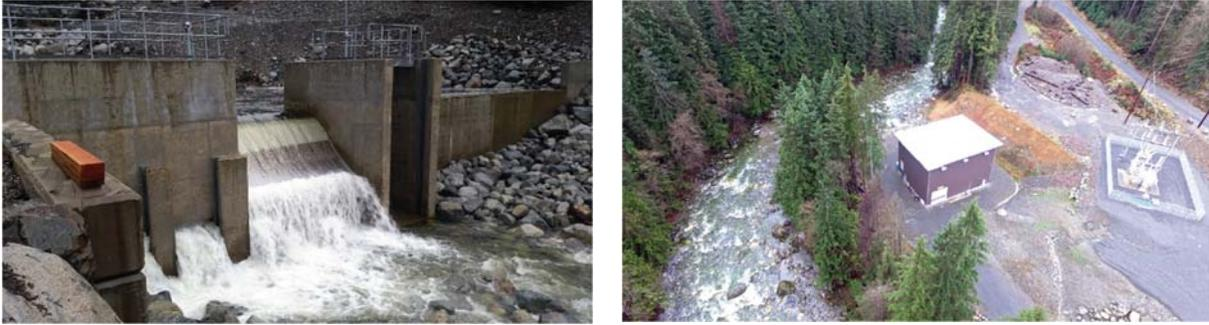
**Figure 1: Marty Creek intake (left) showing the Coanda screen intake and side-spill weirs. Powerhouse and substation (right) adjacent to McNab Creek.**
