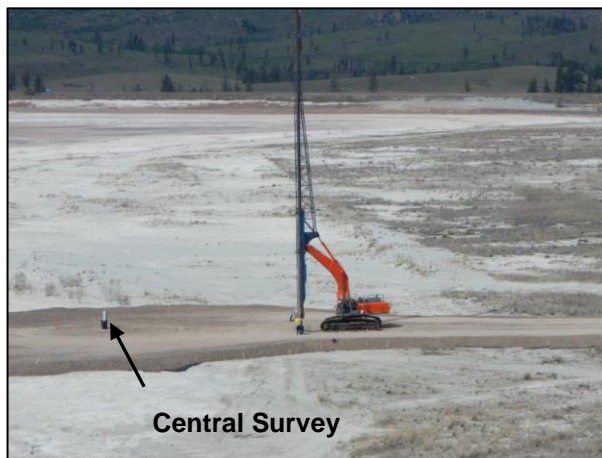
A - Installation of Wick Drains
