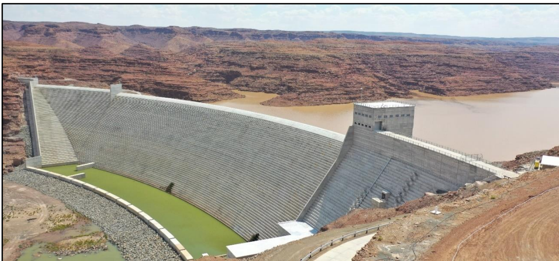
Figure 1. Neckartal Dam view from downstream.
