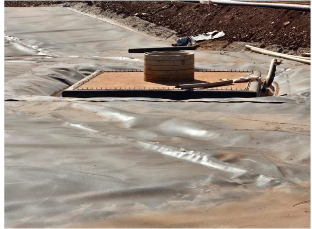
Fig. 1. HPDE geomembrane excess around a fixed structure allowing for settlements.
