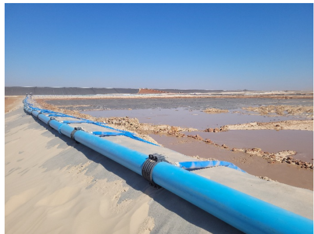
Fig. 2. Hydraulic deposition of tailings over a geomembrane
