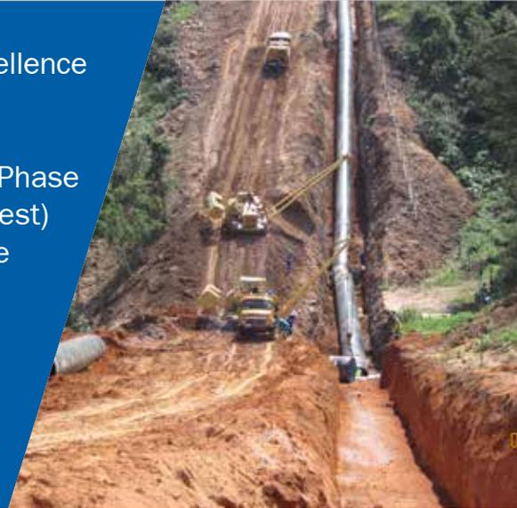
**S**erving the growing needs of the City of eThekweni's industrial and residential sectors is an expanding network of steel pipelines that traverse the hilly terrain common in this region. The challenging topography calls for innovative design and construction methodologies, which had a direct bearing on the pipeline reticulation system adopted.
