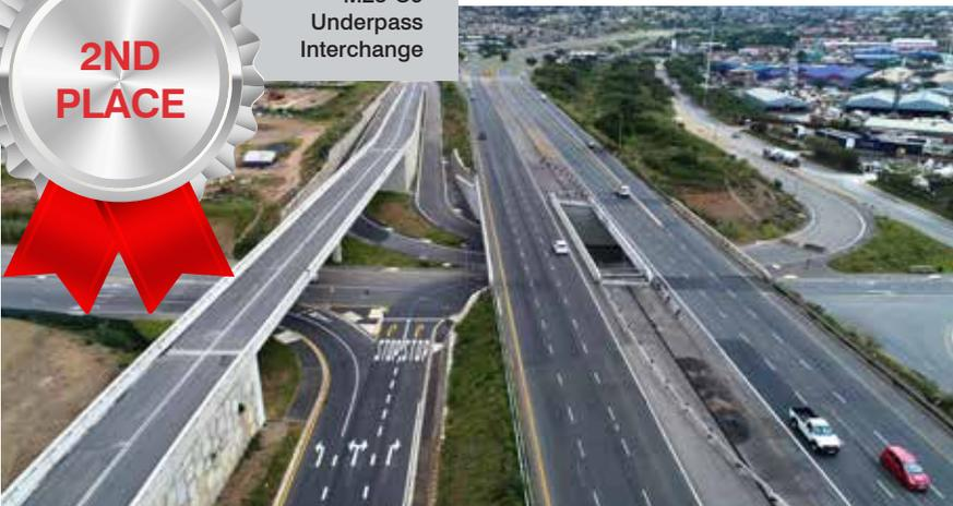
the C9 route to split away smoothly from the C3 route and loop back on itself, a viaduct for the continuing C3 route, realignment of an existing highway off-ramp and creation of a matching on-ramp, and, of course, the underpass itself, which connected the two highway ramps in a half-diamond configuration.
