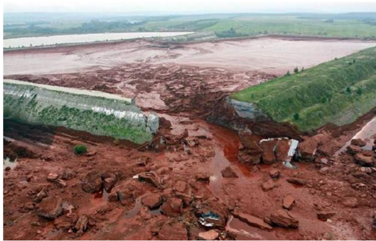
Figure 3. Cone of depression visible after the failure of the Kolontár dam (Oszvald, 2015 in Martin et al., 2015)
