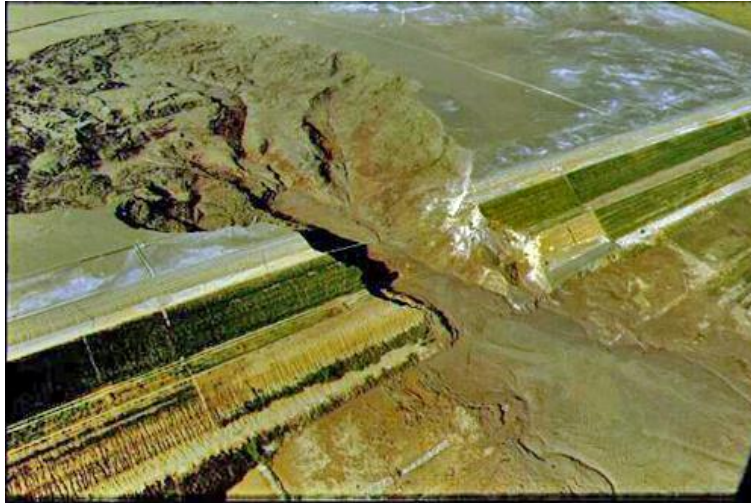
Figure 2. Aerial view indicating the cone of depression after the failure of the Merriespruit TSF in 1994 (Engels, n.d.)
