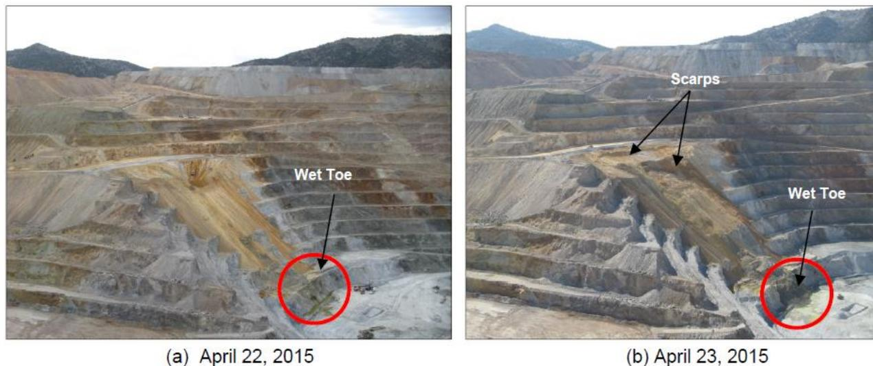
Figure 3. Failure of the east wall.
