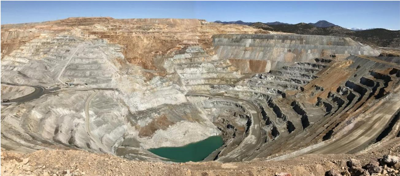
Figure 1. Failure of the north wall (picture taken in early 2017).
