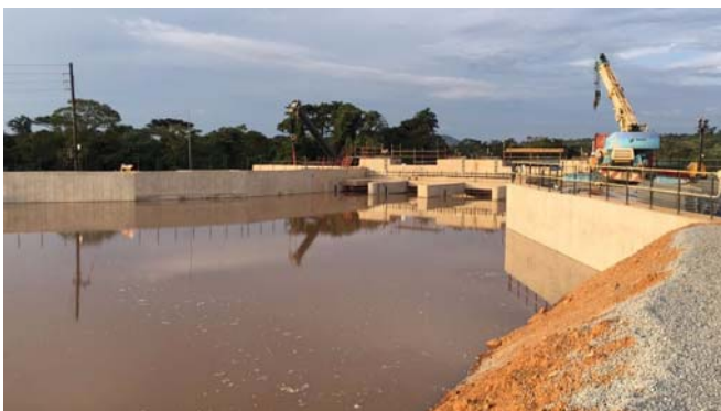
Figure 14: Powerhouse Forebay
