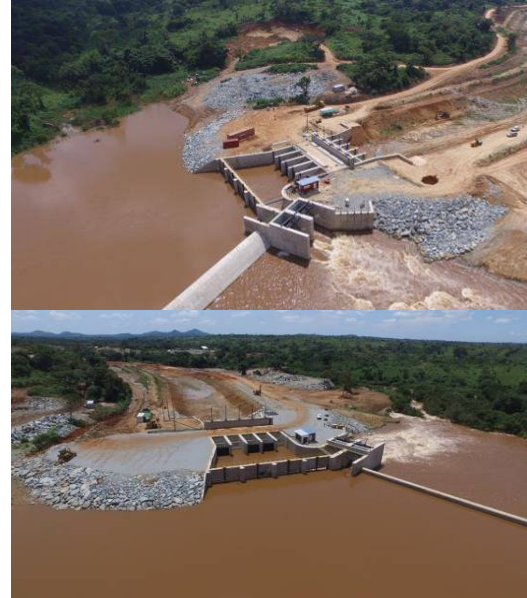
Figure 8: View of Intake Structure
