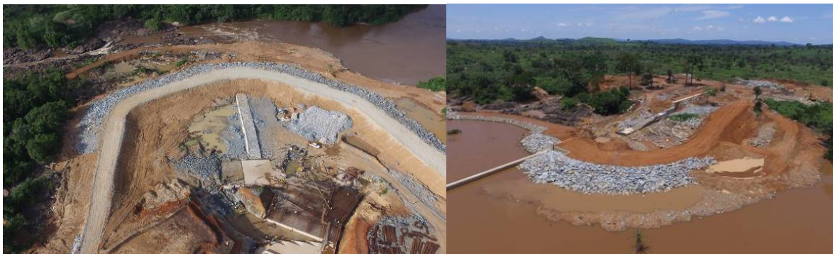
Figure 9: 1 st and 2 nd Stage River Diversion
