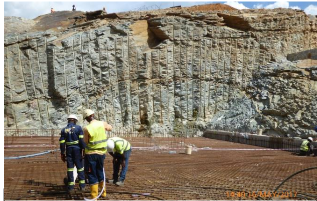
Figure 10: Precision Blasting for Powerhouse
