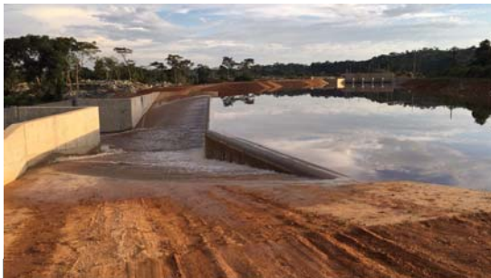
Figure 11: Emergency Spillway
