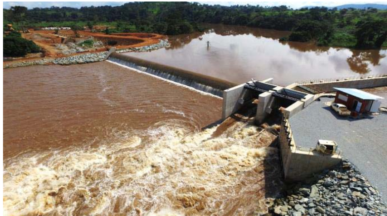
Figure 13: Project headworks viewed from downstream
