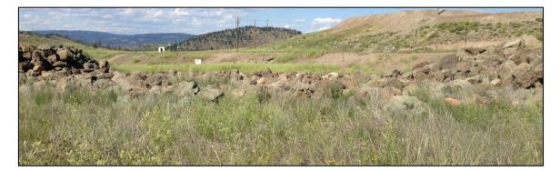
Figure 2. Riprap lined spillway entrance with reclaimed tailings beach in the foreground and waste rock dump on the right side of the frame; looking downstream (northeast)
