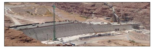
Figure 2. RCC on 7 steps during the construction of the dam wall
