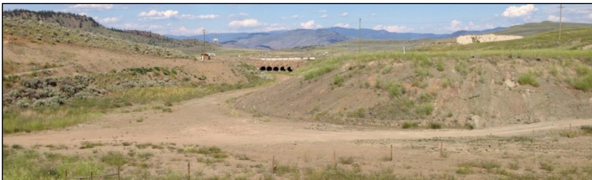
Figure 5: Spillway channel with roadway crossing in background, looking downstream (northeast)
