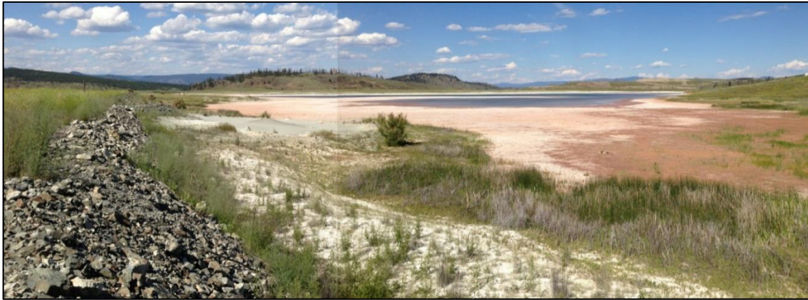
Figure 7: TSF pond on July 9, 2013, looking northeast.
