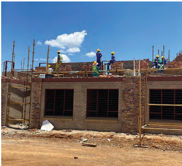
Superstructure brickwork and installation of window and door frames
