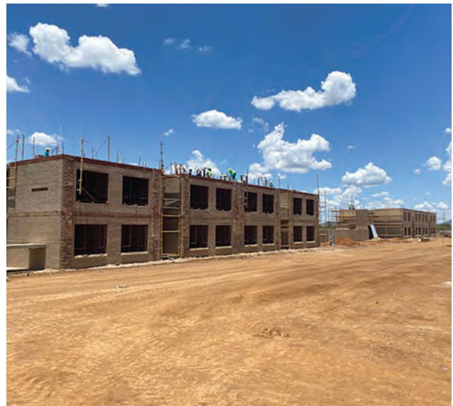
Road-bed layer works compacted and completed and side view of first floors.
