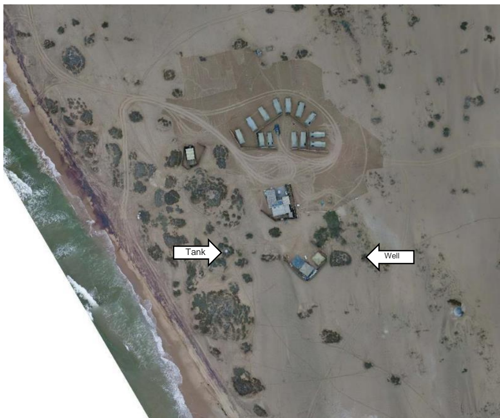
Figure 5: An aerial view of the existing tented camp
